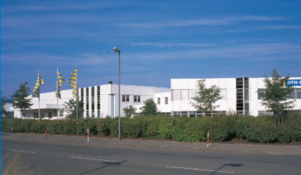
German production facility in Bielefeld
