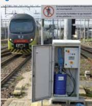
The TRACK-LUBE system has been created to lubricate the rail curve and reduce wear on the wheel as well as on the rail itself.
