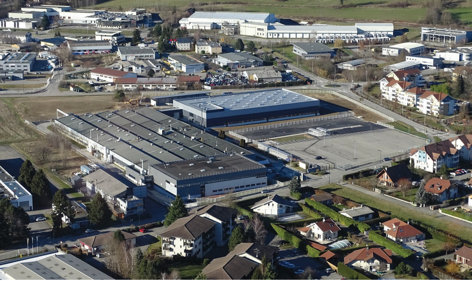
The factory of Argonay and the new building
